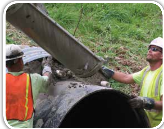
Cast in place headwall
