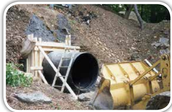
Cast in place headwall
