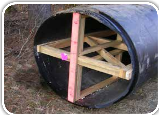
Oval Snap-Tite Pipe® with struts inside, before installation.
