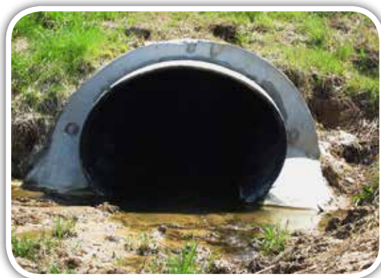
A culvert, rehabilitated with Snap-Tite® oval pipe.
