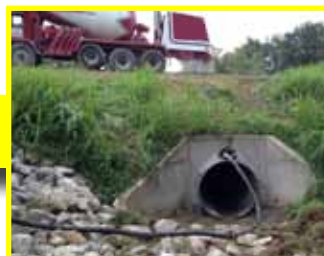
The grout is pumped into the entire length of the pipe, filling in the annular space between the new and host pipe, and the voids outside of the host pipe.
