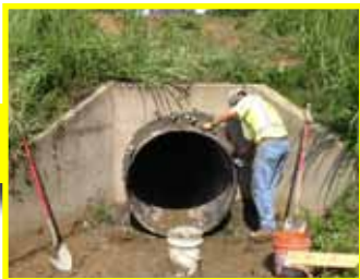
Different length PVC pipe that will deliver the grout flow are installed, and both ends are sealed using concrete bulkheads
