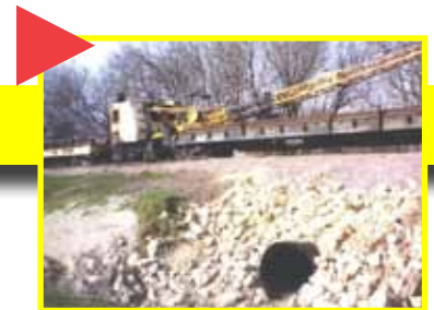
The totally rehabbed Snap-Tite culvert. Nearly all the work was completed off-track in the culvert itself.
