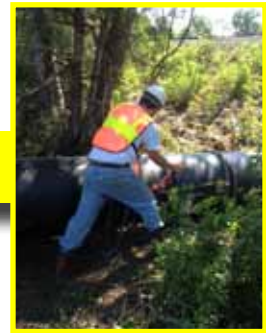
Using chains and pressure from the excavator, the two pieces of pipe are 'snapped' together. The process is repeated until connected sections of Snap-Tite are pushed through the entire length of the culvert.
