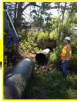
The second piece of pipe is lowered into position, and lined up with the first piece.
