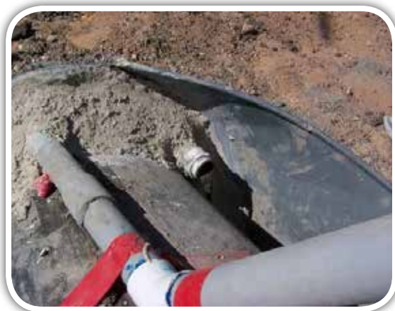
Grout can be seen exiting from the PVC port
