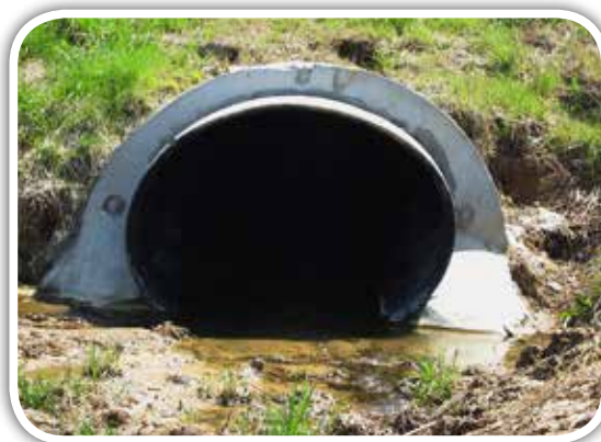
A culvert, rehabilitated with Snap-Tite® oval pipe.
