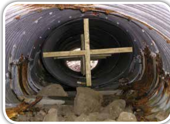
Snap-Tite® pipe coming through a deteriorating culvert during installation (struts will be removed once completed).
